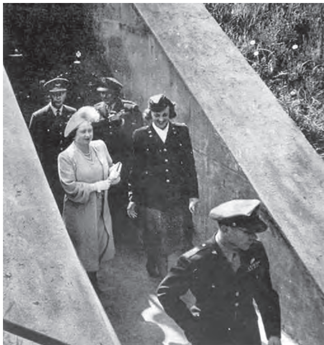
On 11 May 1945 King George VI and Queen Elizabeth visited the bunker at Daws Hill. The King is seen behind the Queen speaking to General James H Doolittle. This is the 'wartime' entrance to the bunker. It's now the emergency exit and equipment entrance.
